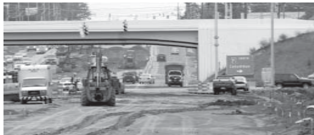
Work on State Route 18 at Interstate 71 in Medina Co.
