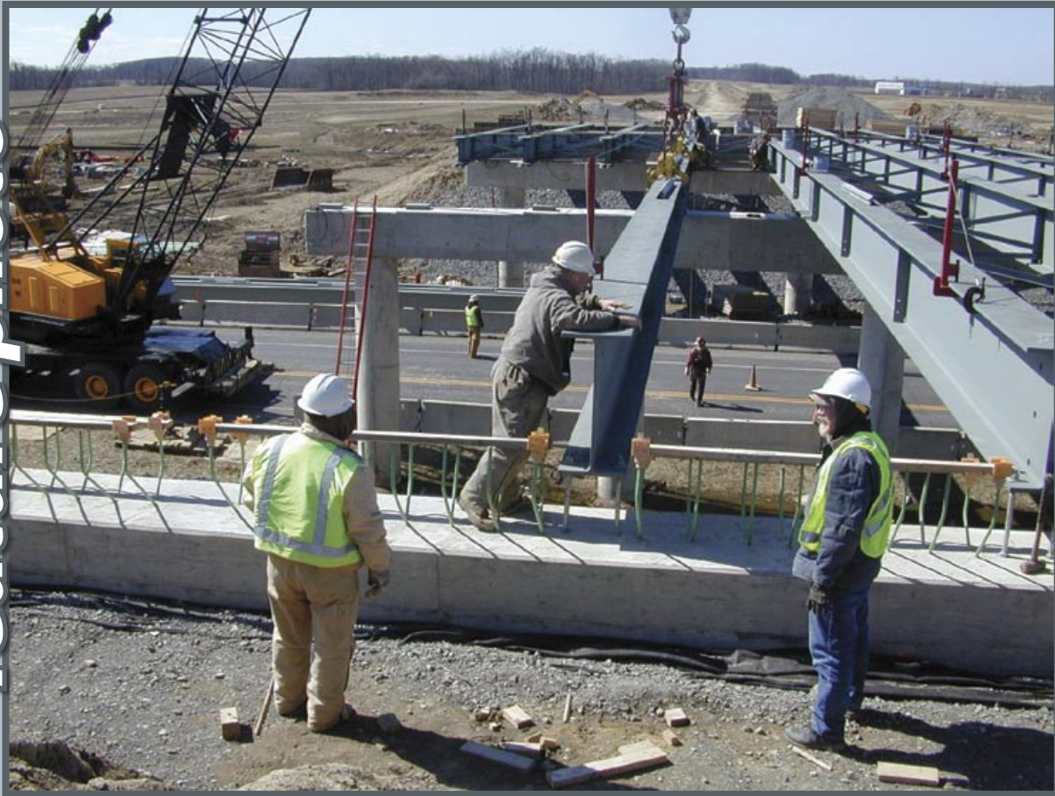
Beams being set for the new U.S. Route 30 over U.S. Route 68 near Williamstown, Hancock County in March 2006. The rough grade of the new U.S. 30 highway alignment is visible in the background stretching to the west.
