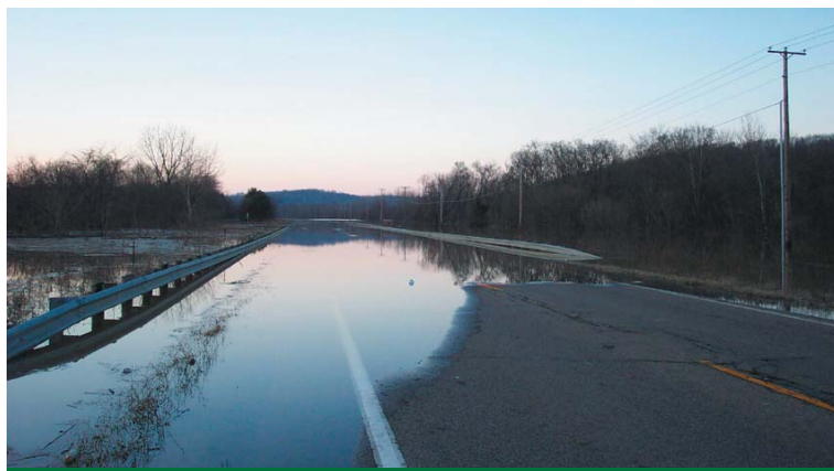
Flooding on State Route 60 and Pioneer Drive in Muskingum County.
